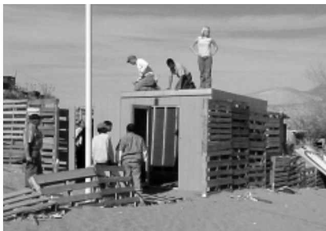
Ben and other volunteers doing some much needed repairs.
